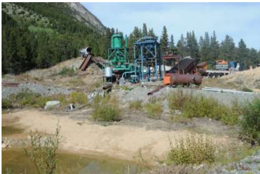
Figure 34. Small gold mine ore concentrator and tailings pond (foreground) at Pellaire mine camp, Falls Creek. The mine site is currently in a state of abandonment and the tailings pond may be leaching contaminants into a small creek that runs into Falls River. Fuel storage barrels and mine chemical barrels also have been left to the elements.
